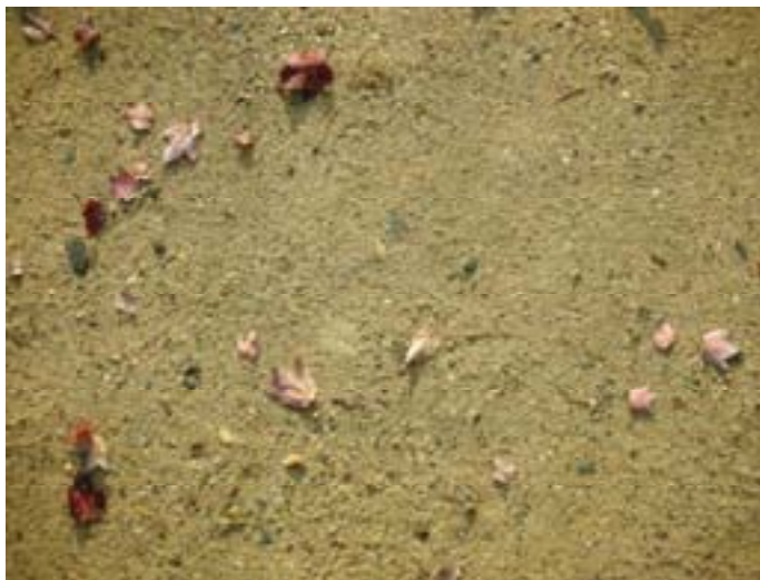
Figure 3. View of the sand like surface. The path is compacted stone dust and does not show bike tracks or foot prints. Minute Man National Park (Concord).
