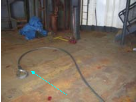
Replaced deck plate
