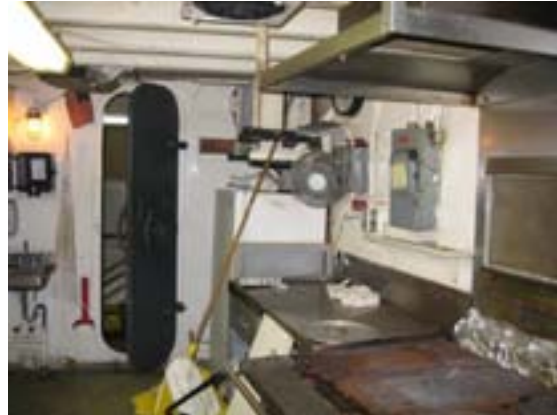
Water tight door
