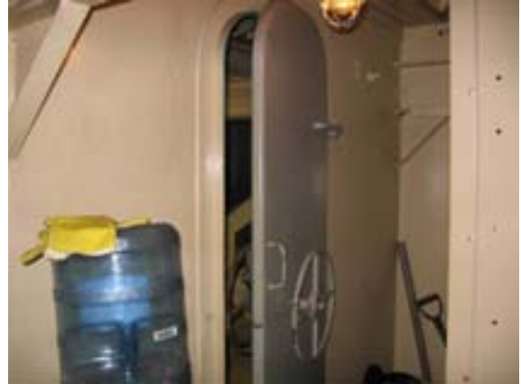
Watertight door in Bulkhead #36 aft
