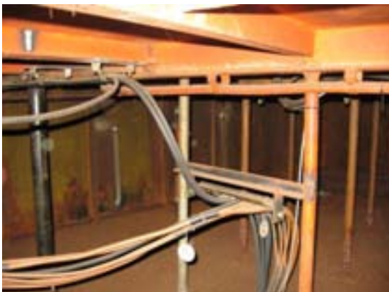
Void space under wheelhouse
