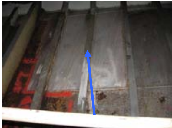
Replaced plate in shell
