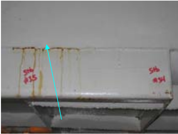
Cracked Welds
