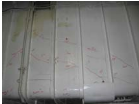
Buckled bulkhead - port midship
