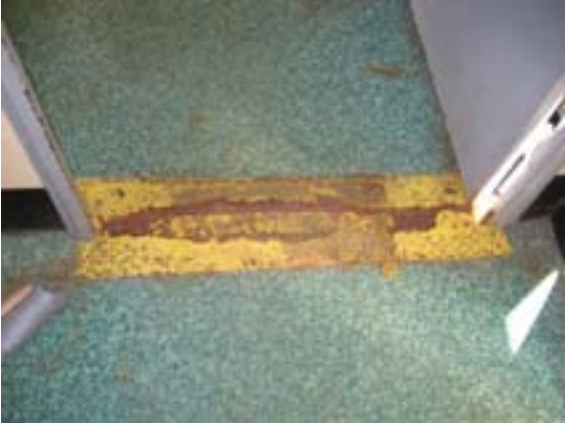
Wasted threshold
