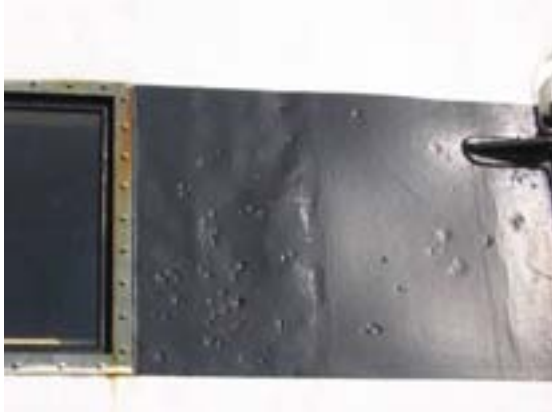
Pitting in superstructure
