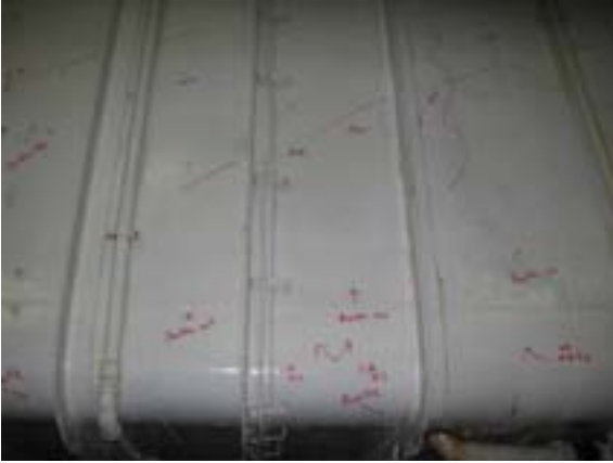
Buckled bulkhead - starboard midship
