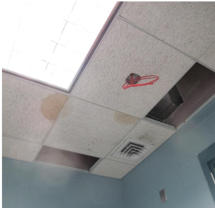
Dirt pattern on DCTs indicating ineffective air filter for air handler serving Briefing Room
