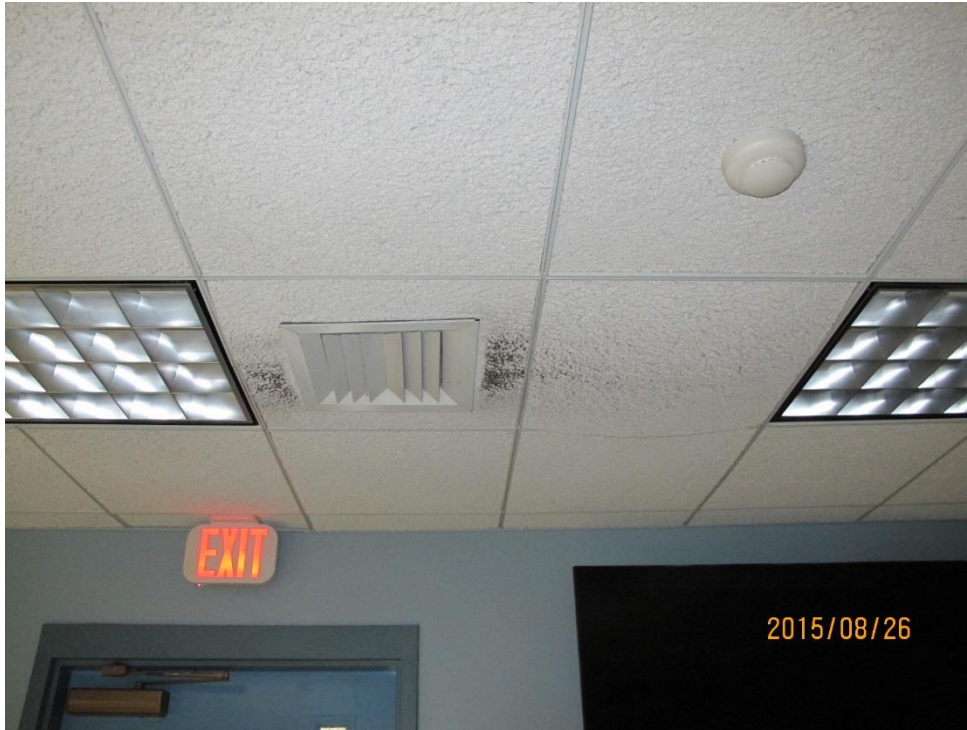
Dirt pattern on DCTs indicating ineffective air filter for air handler serving Briefing Room
