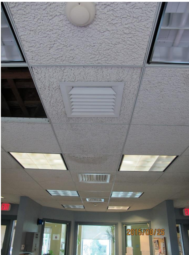
Clean supply grates in reception area
