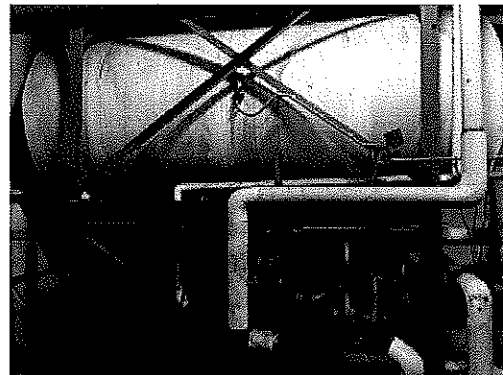
1957 Building Indirect Domestic Hot Water Tank
